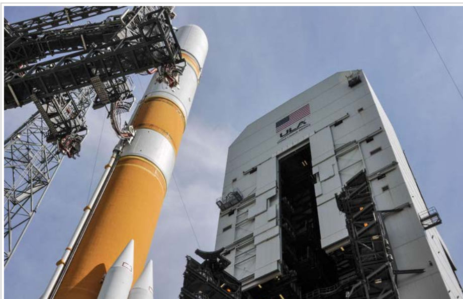
The Mobile Service Tower is rolled back at Space Launch Complex 37 in preparation for launch of the Air Force's sixth Wideband Global SATCOM satellite. (Photo: United Launch Alliance, LLC)
