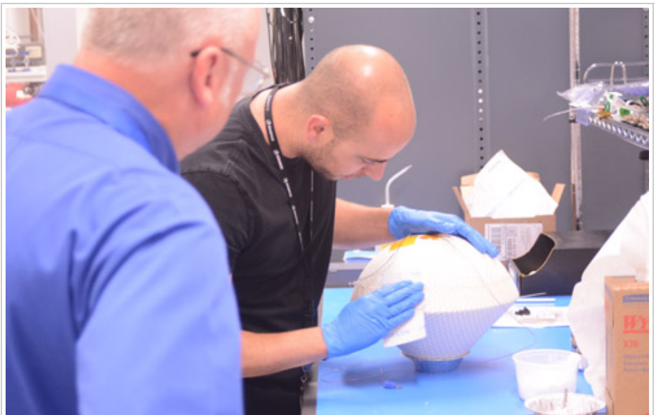
Geoff Maul sands excess sealing compound from the REBR-W heat shield on Nov. 11. At left is Nathan Harnagel from the Aerospace Houston office. (Photo: Dave Hinkley)
